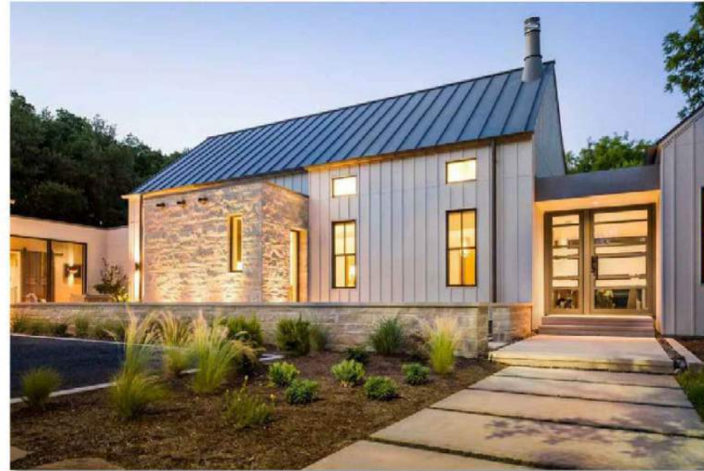
Standing Seam Metal Roof
