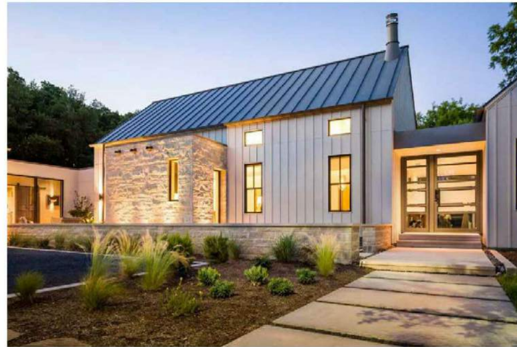
Standing Seam Metal Roof
